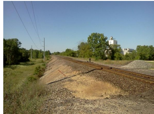
Rail line crossing at Packard Highway.
