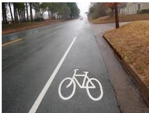
Example of dedicated bike lane.
