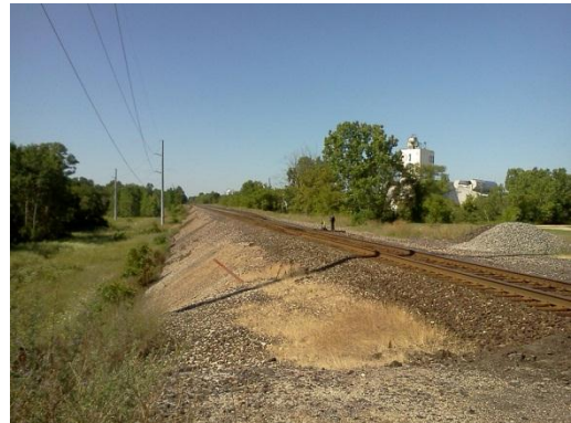
Rail line crossing at Packard Highway.
