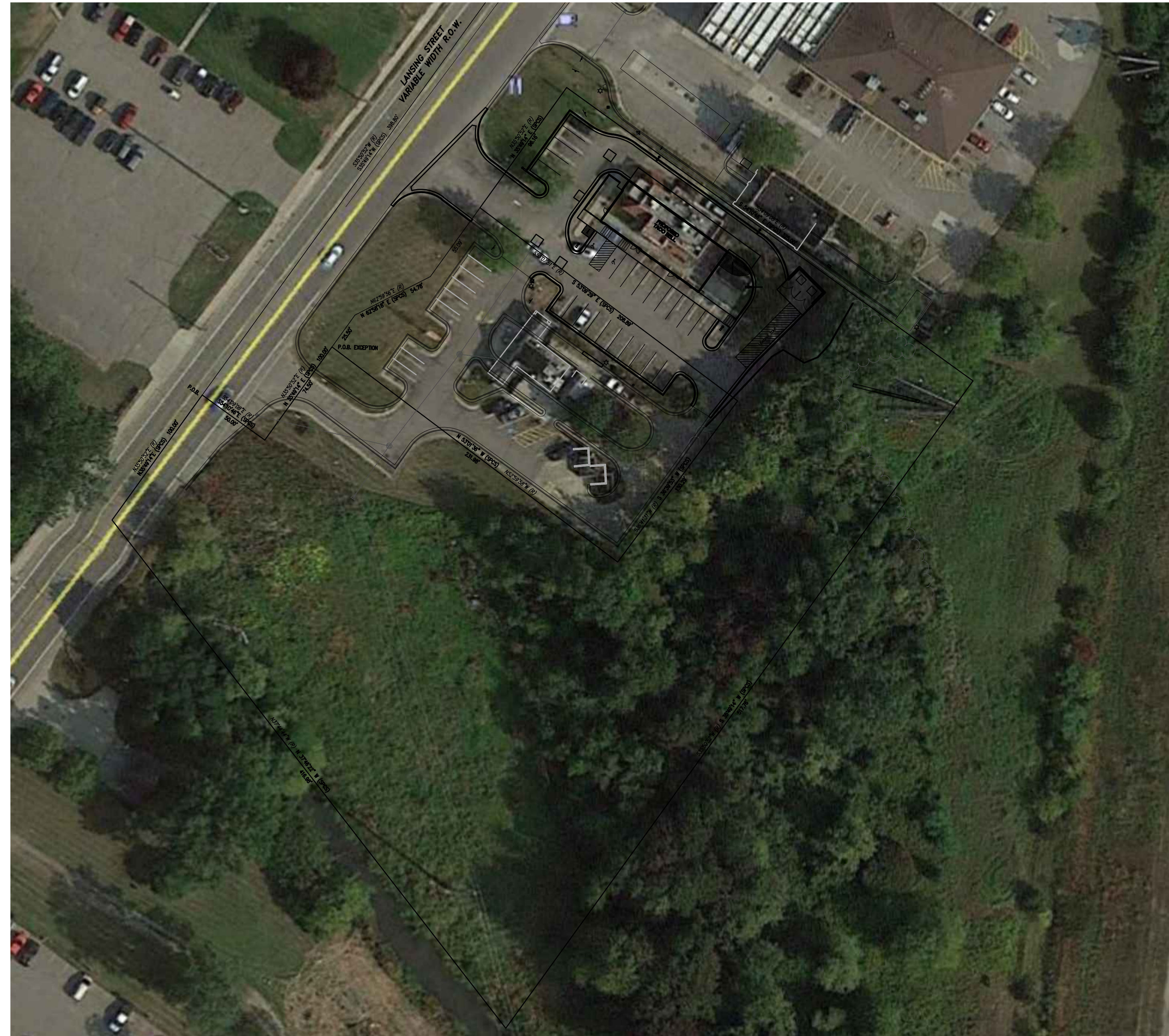
AERIAL PHOTOGRAPH SCALE: 1 IN = 50 FT
