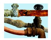
Part of that work includes verifying the material of the water service inside the residence. Water service lines can be copper or plastic, but some may be galvanized steel, iron, or lead.
